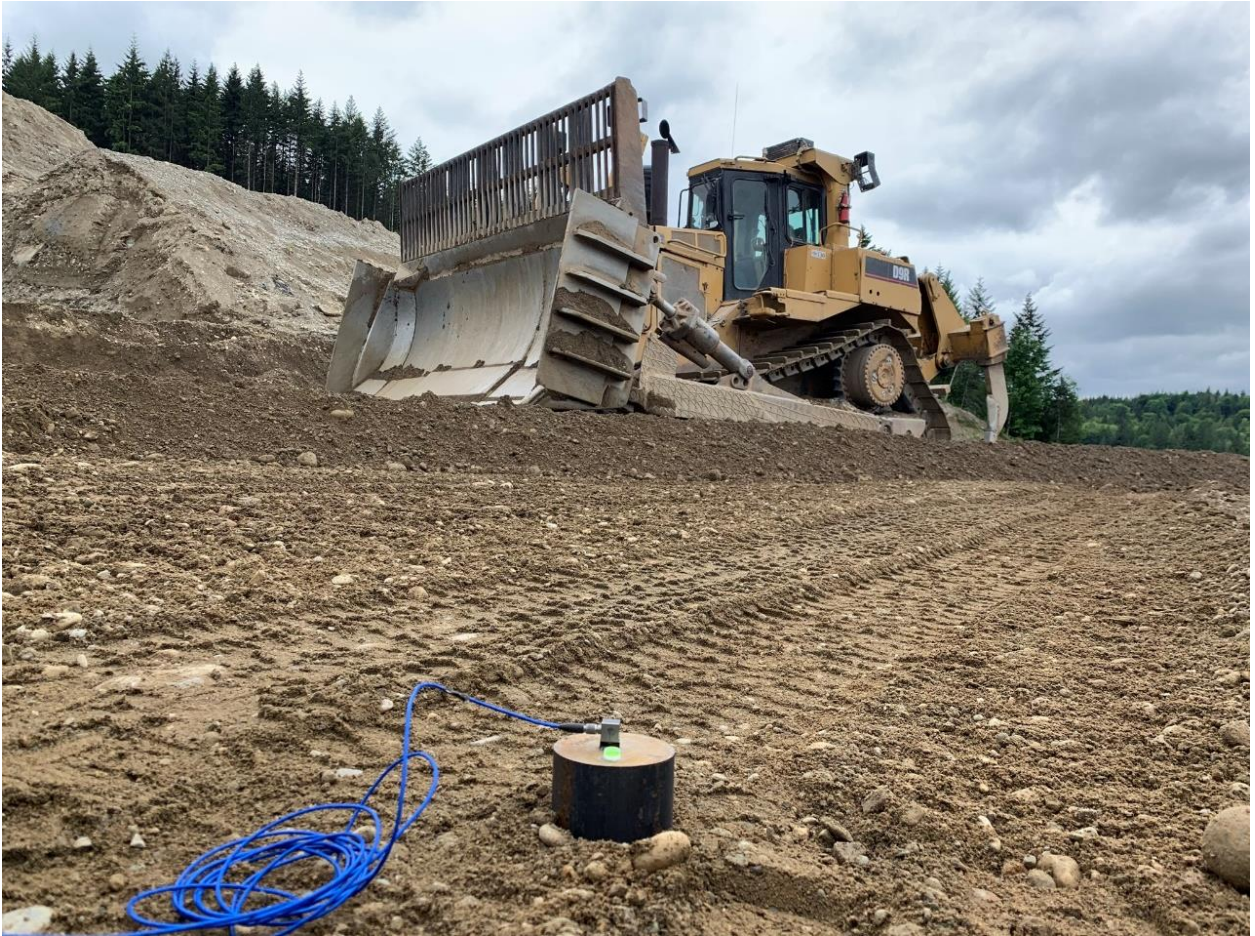
Figure D1. Typical Vibration Measurement Setup
